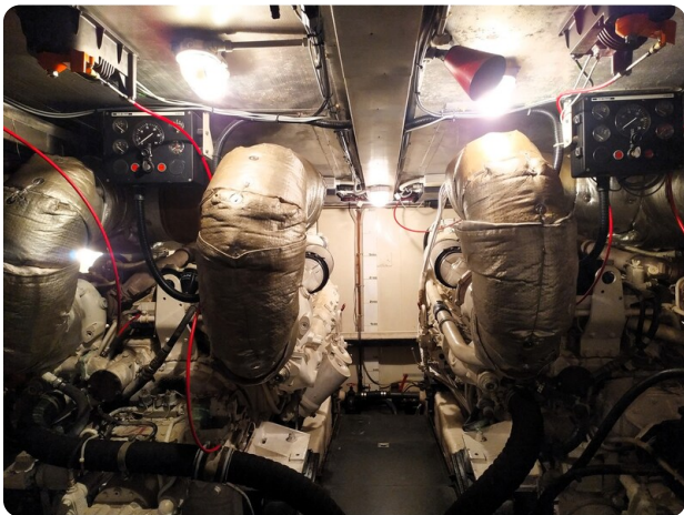
SANLORENZO SL 62 Engine Room
